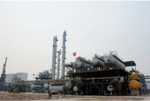
20 万吨/年离子液体协同催化烷基化生产汽油添加剂 Industrial production line of alkylation oil by using ILs as the promoter instead of sulfuric acid (capacity: 200,000 tons/a)
