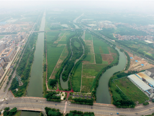
东莞燕岭湿地生态园人工湿地工程 Constructed wetland project of Dongguan Yanling wetland ecological park
